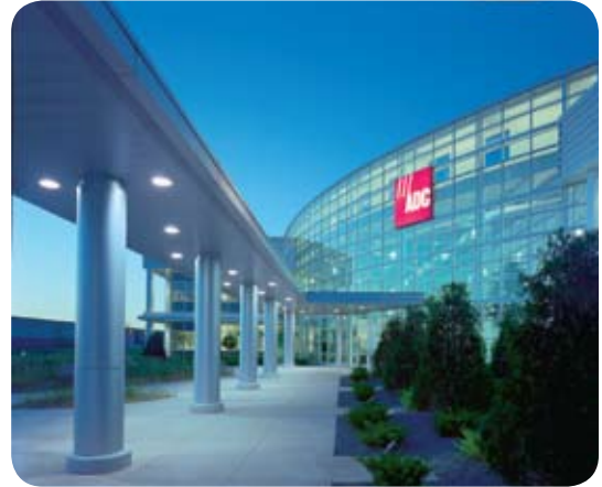
ADC's state-of-the-art facility in Shakopee, MN
