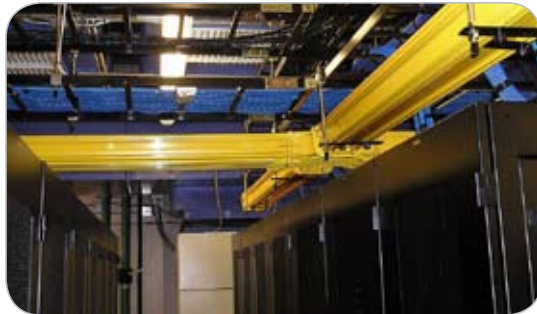
ADC's FiberGuide® – Ensuring proper bend radius and ultimate fiber protection
